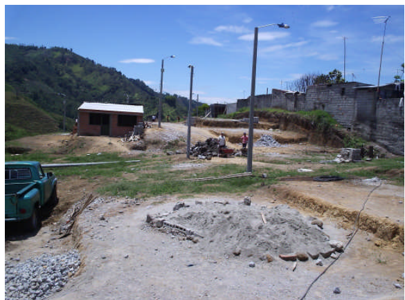
The Electric Light Posts Are Now In Place
