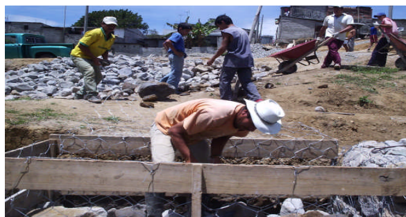
Building Retaining Wall With Manual Labor
