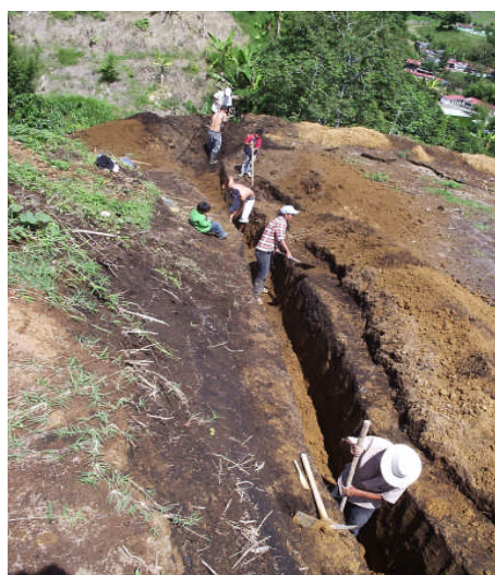
Putting In The Sewer Lines
