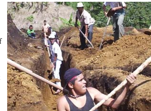
GROUND BROKEN ON OUR HOUSING PROJECT IN SOUTH AMERICA
