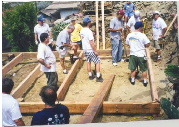
Laying The Foundation
